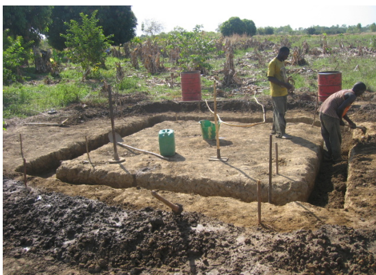
Pond construction in Bougouni (Seydou Toé).
