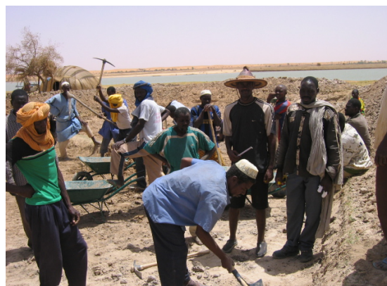
Pond construction in Gao (Seydou Toé).
